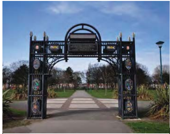
Figure 6: Entrance into Ayresome Gardens
