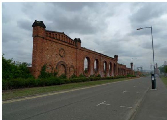
Grade 2 listed wall on Vulcan Street
