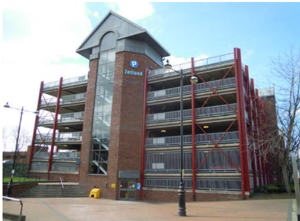
The Zetland multi-storey car park, accessed from Station Street
