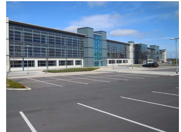
Business Park-type approaches to parking should only be considered in parts of the study area where access by non-car modes is poor.
