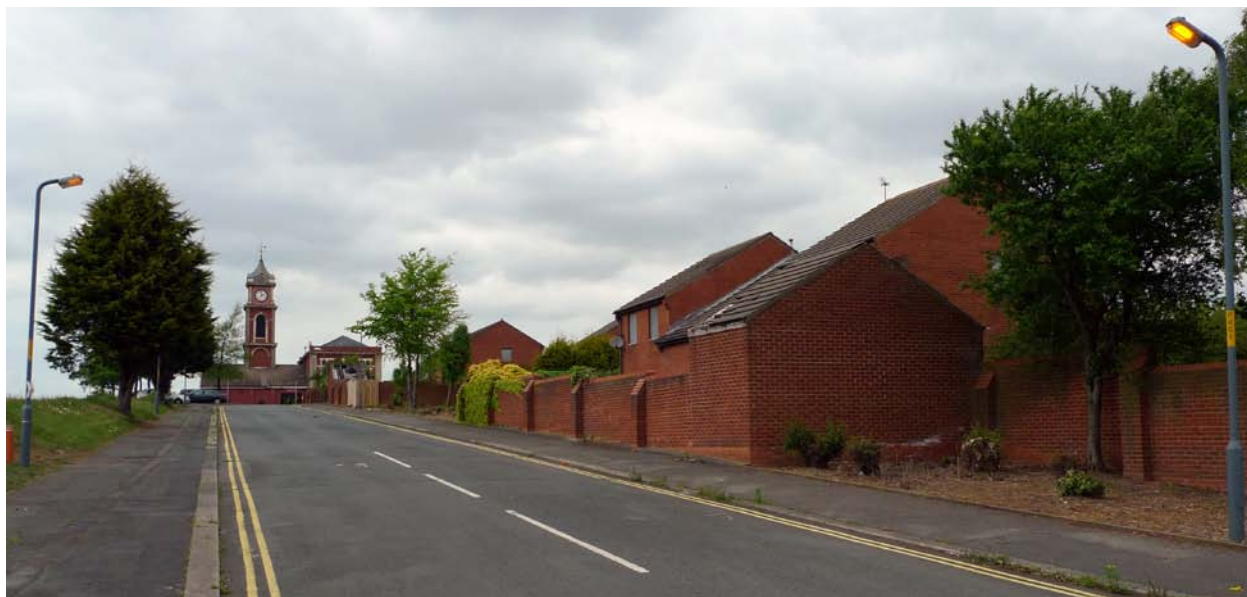
The derelict Old Town Hall and remains of the St. Hilda's housing estate
