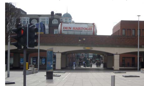
The Zetland link looking south, with the A66 above.
