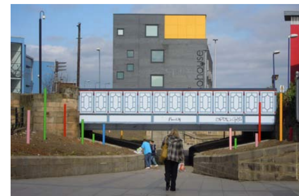
The Zetland link looking north, with the railway bridge above.
