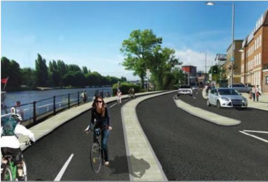
Complete segregation of cycles and vehicles adjacent to carriageway(main roads – Marton/Acklam/Ormesby/Cargo Fleet Lane)
